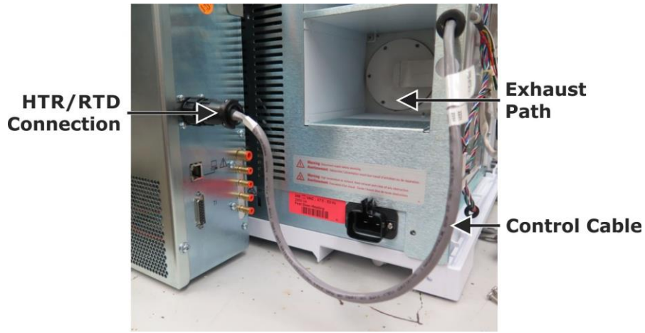
Figure 3-46 Control Cable Installed to 7890 Control Box
